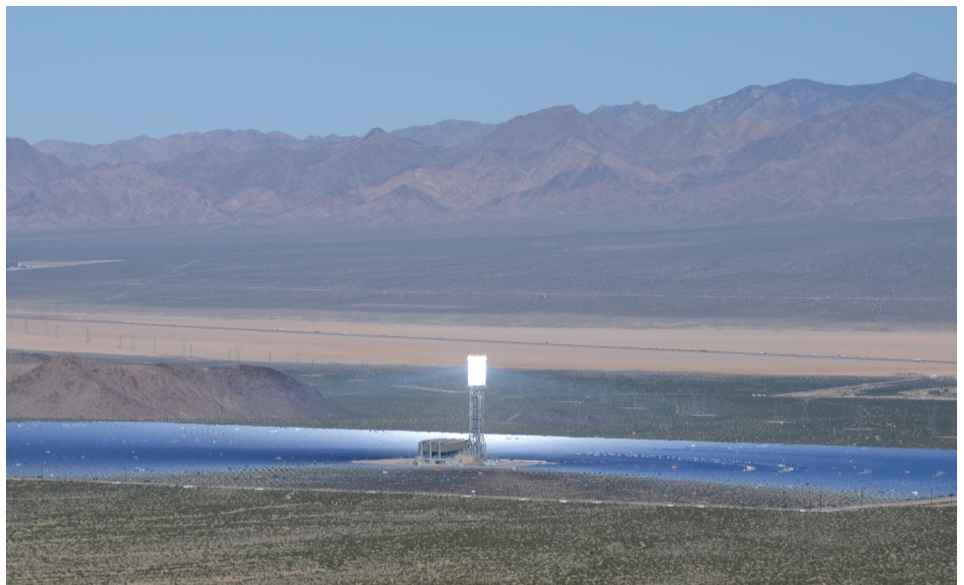
Ivanpah Solar Electric Generating System (Photo credit: R. Sullivan, Argonne National Laboratory)
