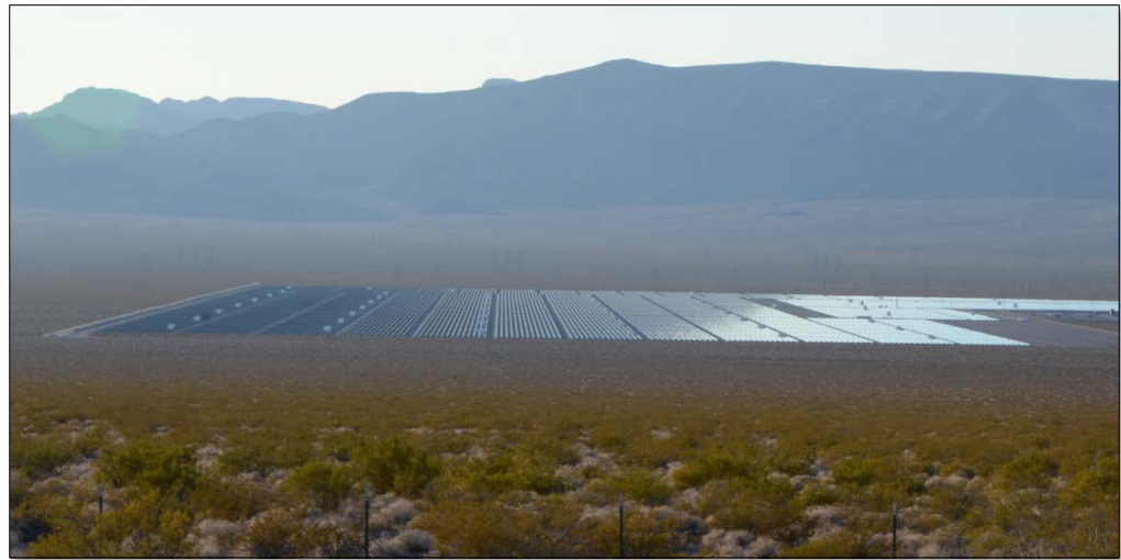
Copper Mountain Solar Facility, Boulder City, Nevada. (Photo credit: R. Sullivan, Argonne National Laboratory)
