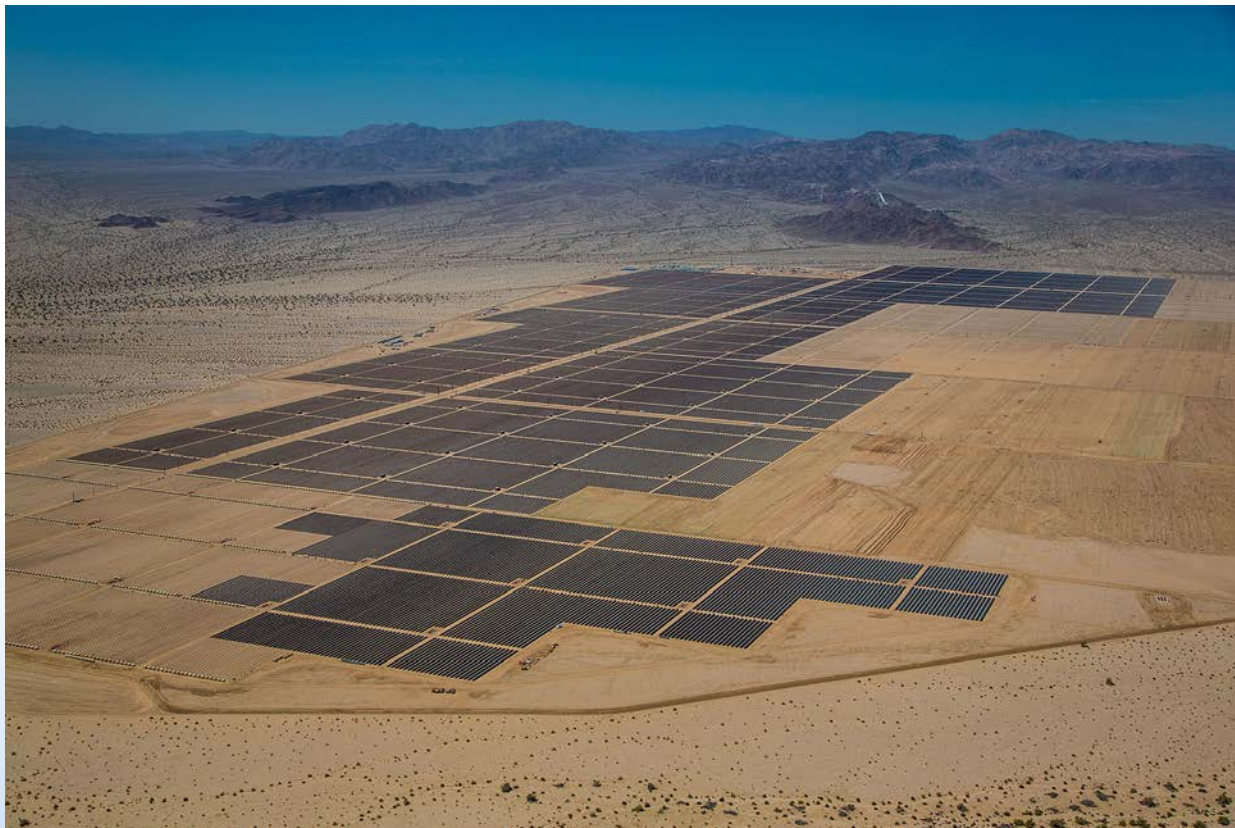
Desert Sunlight 550 MW Photovoltaic Facility
