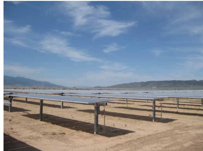
Scatec Solar, Iron County, Utah
